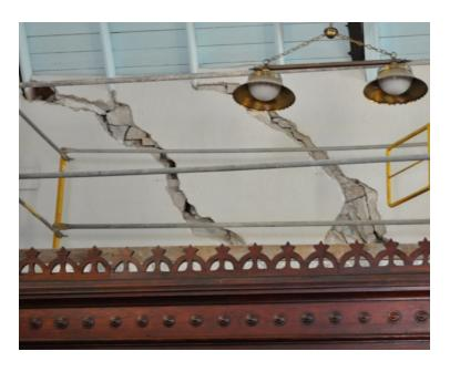
Jack Newsom took this great picture of the inside of our church. It shows the corner above the choir loft. You can see Where the plaster has been removed to expose a rock wall. We learned that our church walls are actually composed of 2 layers of rock. The exterior rock wall is mortared together while this interior wall consists of rocks that are simply balanced on one another!!
